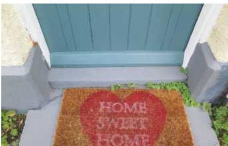
PIC 11. Weatherboard fitted and sealed to the door with silicone
