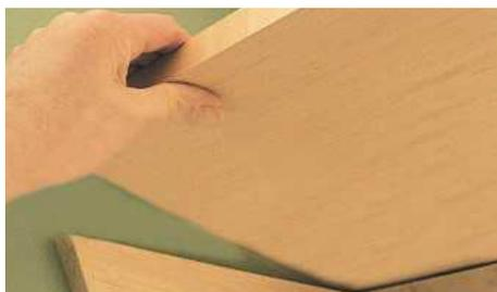
**STEP 19.** You'll probably need to trim the shelf ends with a plane to get it to fit the alcove neatly. Don't force it, as this could split veneer or damage plaster
