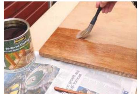
**STEP 6.** To restrict a plastic container from sliding, brush on a couple of coats of a suitable textured decking oil or paint
