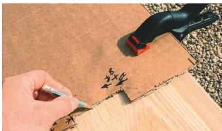
**STEP 16.** Once the template fits nicely, cramp it to the board and draw around the edge. The shelf will be notched out at each end to fit around the beams
