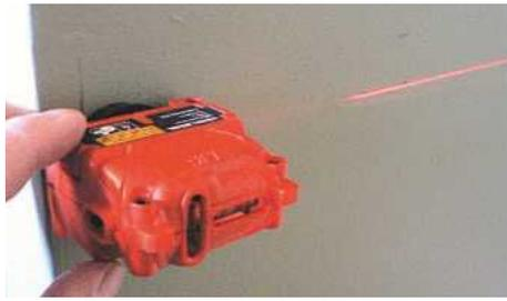
**STEP 7.** A simple laser device will enable you to transfer levels precisely around the room. Use a pencil to mark the lines
