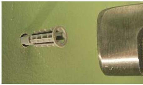
**STEP 10.** Insert a plug in the hole and tap it home. With plastered walls tap slightly beneath the surface, using a large nailpunch or piece of steel rod
