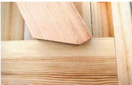
PIC 7. Diagonal brace before marking and cutting into the rail
