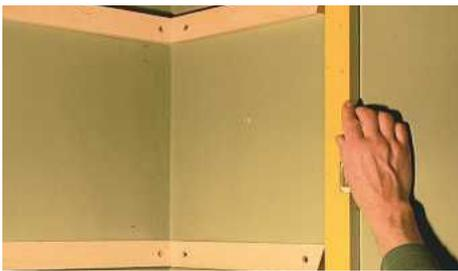
**STEP 12.** When you have several shelves to install above each other, check the side battens line up vertically. Draw a pencil line, then saw battens to fit
