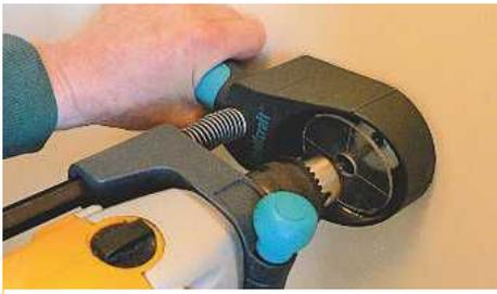
**STEP 9.** It's important to drill holes at 90° to the wall, otherwise you'll struggle to get battens level
