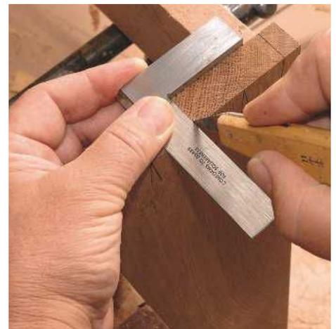
PIC 14. The ends of the tails are marked across the board at right angles
