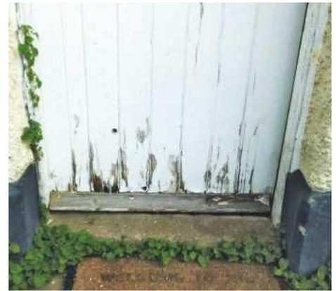
PIC 2. Bottom of door showing extensive rot
