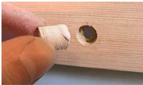
**STEP 13.** Brush PVA on the end of the plug and tap it into the hole, with grain in line with the batten. When dry, saw off the excess
