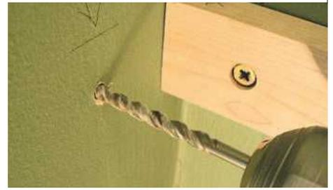
**STEP 8.** Select the correct size drill bit to suit your wall fixing. For holes in brick or concrete a drill with hammer action, plus TCT masonry bit, are essential
