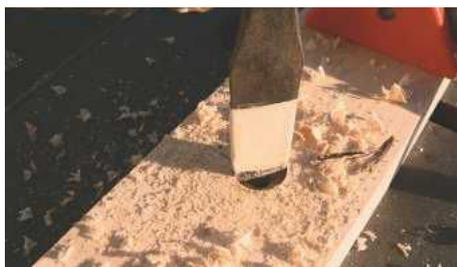
**STEP 4.** Counterbore the screw holes, using masking tape on the flatbit to drill to correct depth. Once the battens are fitted, these holes will be plugged
